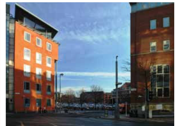
▲ Site as existing from Neville Street
